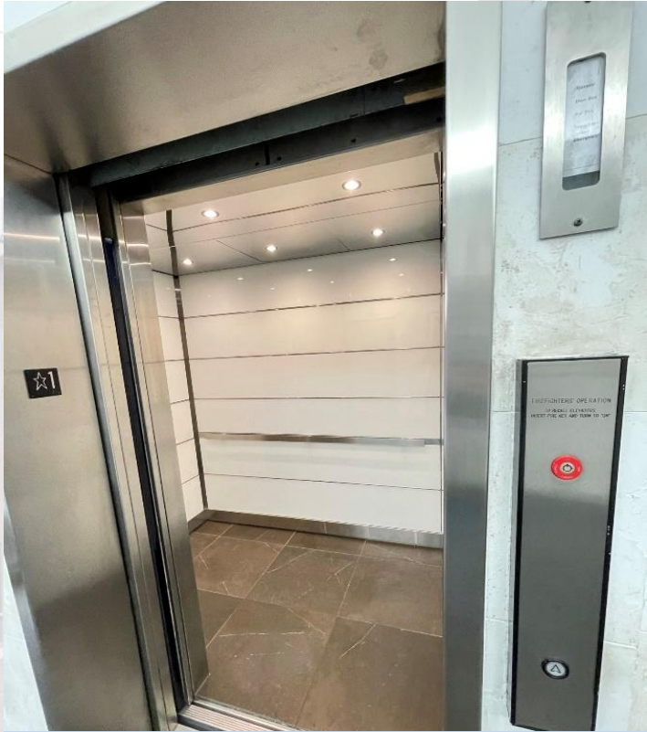
Renovated Elevator Cab
